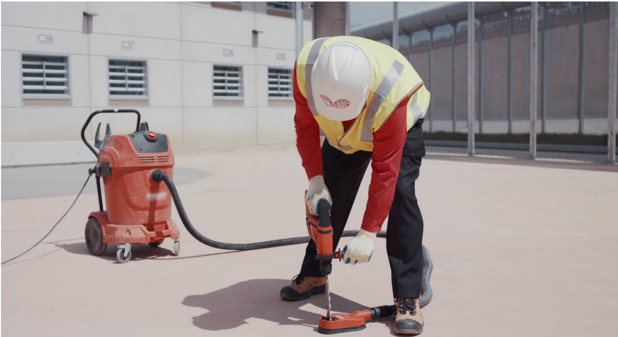
Image 2: Concrete drilling using Hepa filtered vacuum extraction.
