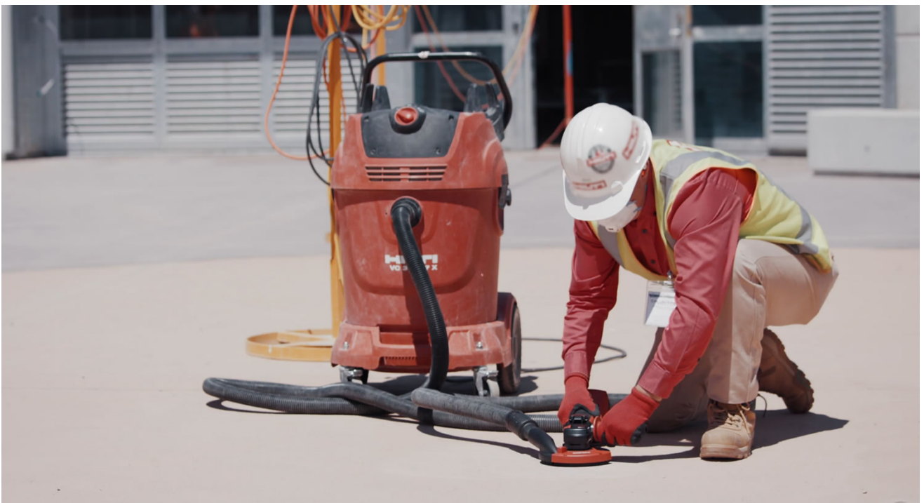
Image 3: Concrete grinding using Hepa filtered vacuum extraction.
