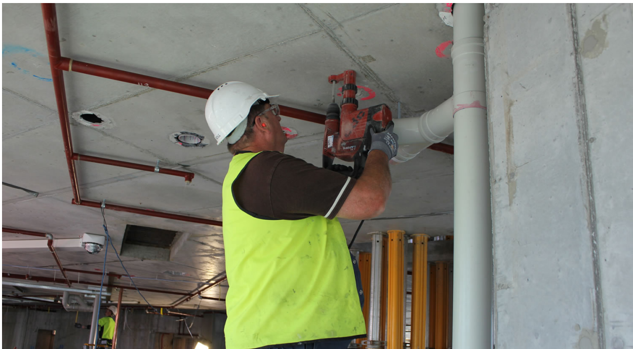
Image 1: Overhead drilling with on-tool dust extraction.
